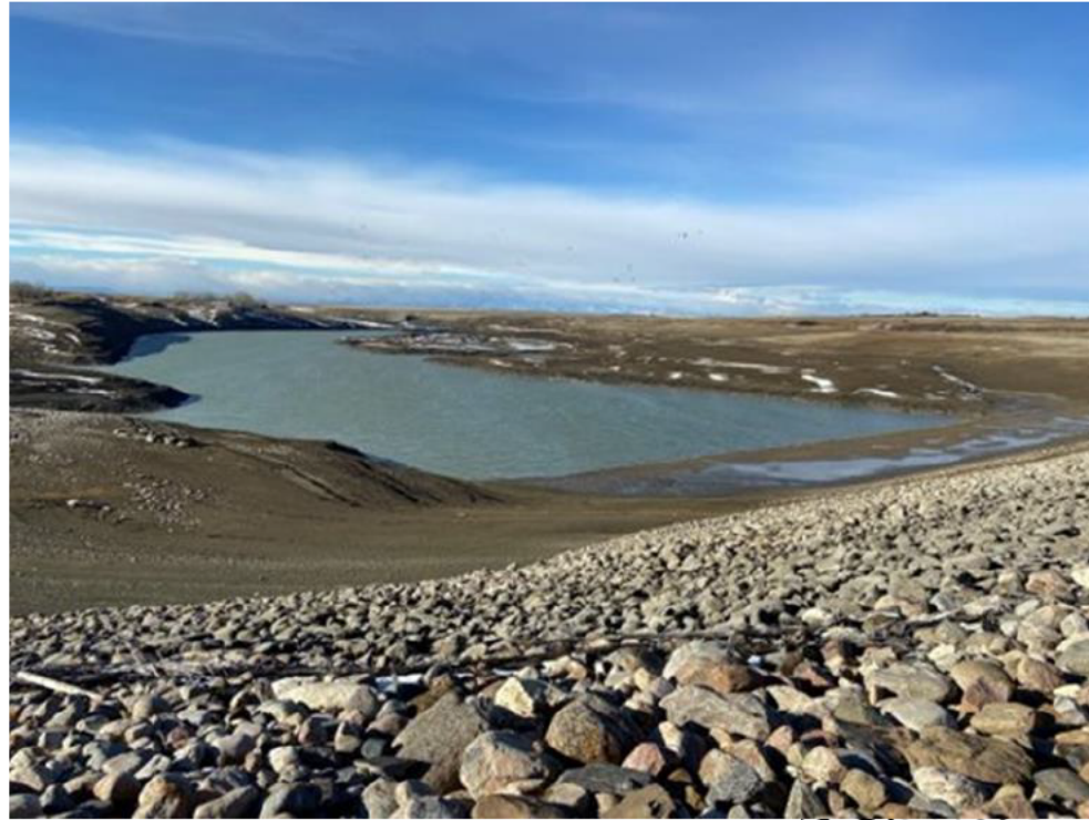
View from the top of the dam
